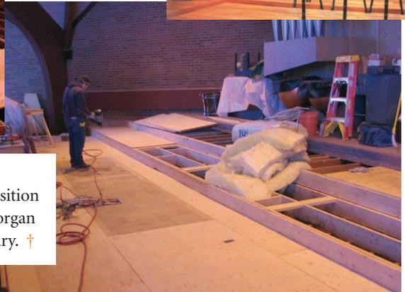
Our organ company disconnected the organ console from the organ case in order to reposition the cables below the floor and to rewire the organ to accommodate the organ pipes from Calvary. †
